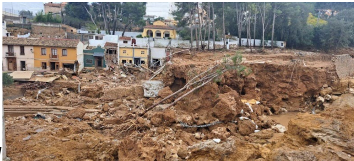
Damages in the Poyo ravine in Chiva
